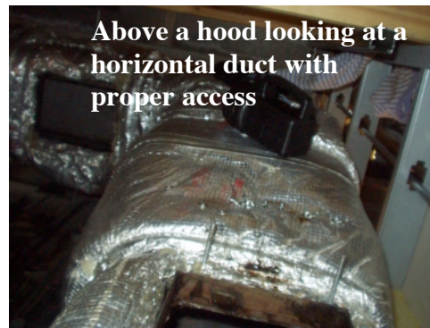
Looking up from the hood into the grease duct, partially inspecting the horizontal plenum area
