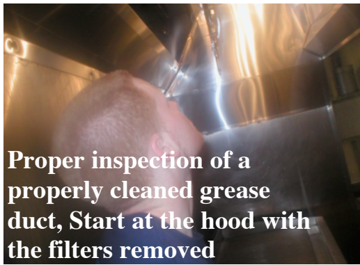
Looking behind the filter rack
