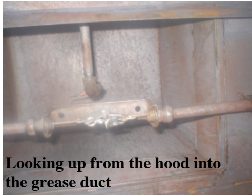
Proper inspection of a properly cleaned grease duct, Start at the hood with the filters removed
