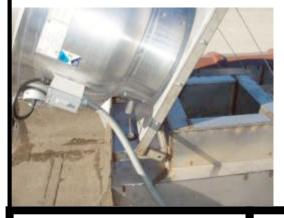
1) Measure the <u>inside</u> of the fan base. We have dimensions for most major fan manufacturers.
